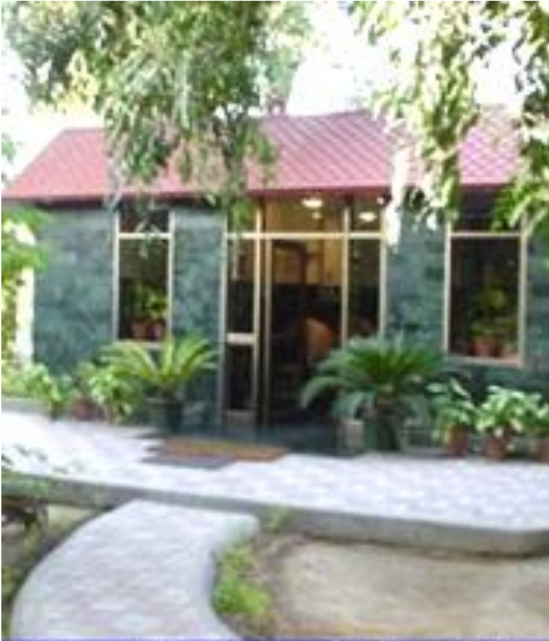
Yes, this is a public toilet
